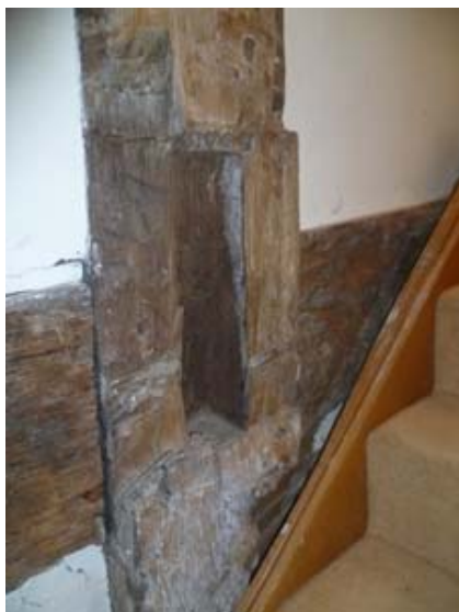
Photo 3: Mortice in front wall post formerly holding the end of one of the hall ceiling's transverse beams
