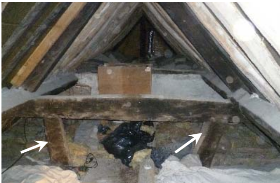
Photo 10: Cores BIWH04 (right) & BIWH05 (left)
