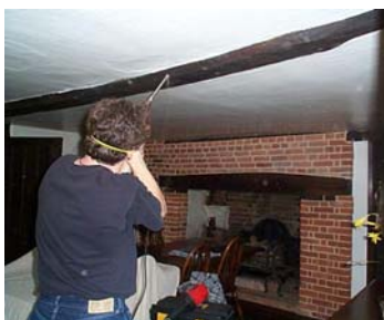
Photo 6: Extraction of a core in progress
